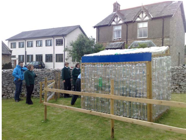
Photo: a Green house made out of plastic bottles in the school yard. ( Courtesy of JDL Giraldo)
